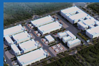
Zhangzhou Industrial Park
