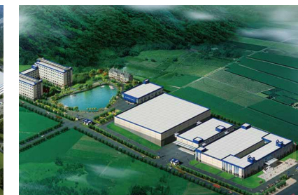
Zhongjiang Industrial Park
