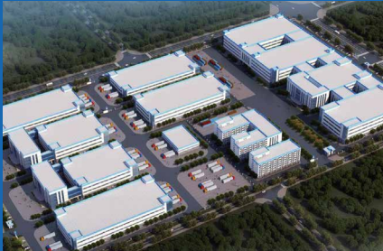
Zhangzhou Industrial Park
