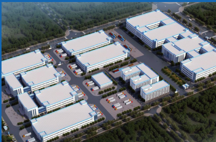
Zhangzhou Industrial Park
