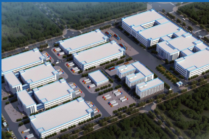
Zhangzhou Industrial Park
