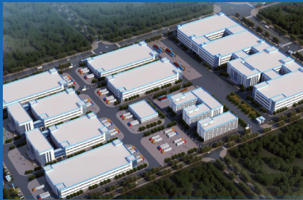
Zhangzhou Industrial Park
