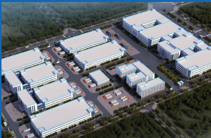
Zhangzhou Industrial Park
